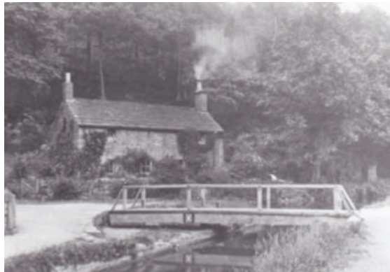
The now-ruined aqueduct cottage at the foot of Lea Wood.
