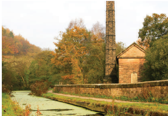
Lea Wood pumphouse on the Cromford Canal.
